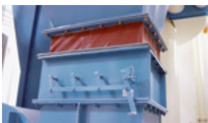
Fabric expansion joint with rectangular flanges
