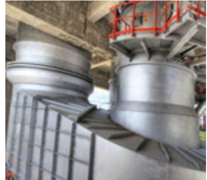
LATERAL EXPANSION JOINT
